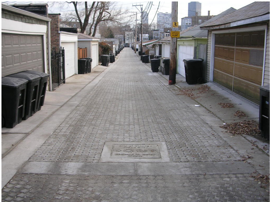
Figure 12 Chicago Green Alley Permeable Paving
